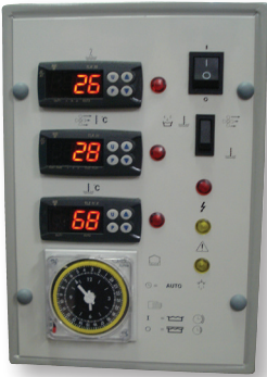
Air and water LPHW control panel
